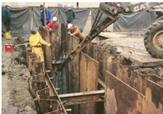
Construction of a PRB in Sunnyvale, CA
